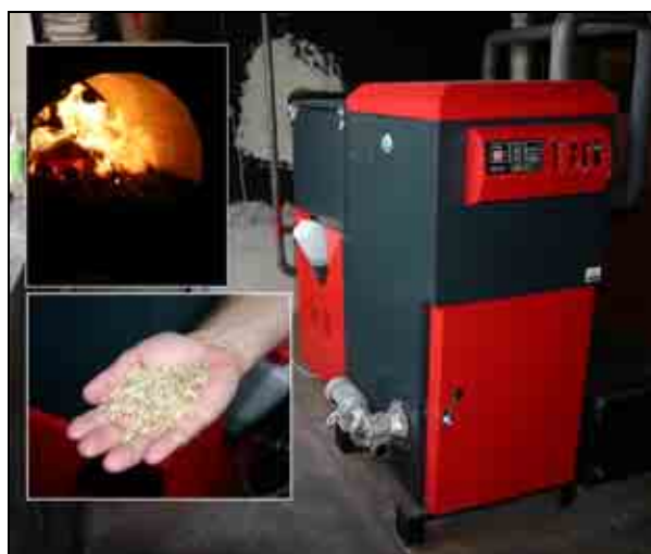
Picture 8 – The example of heat production - the combustion of waste corn in the farm.
